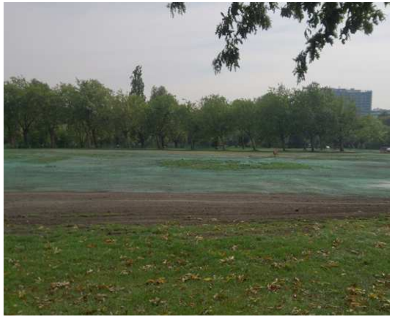
Hard standing following Hydro-seeding (September 2013)
